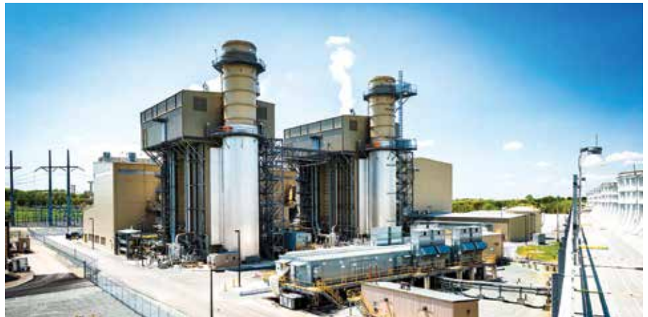
ODEC’s plant in Cecil County, Wildcat Point, provides clean, reliable power for more than 390,000 homes in the region.
