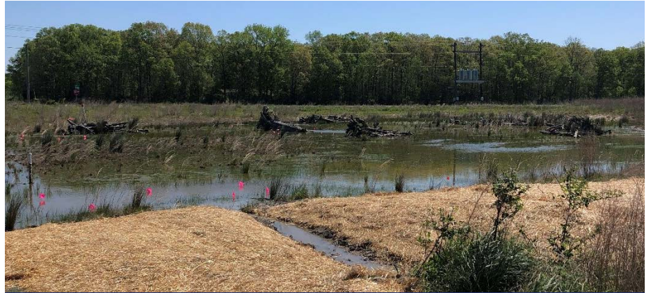
Site conditions as of April 2020, typical in spring with higher water levels before vegetation blooms.
